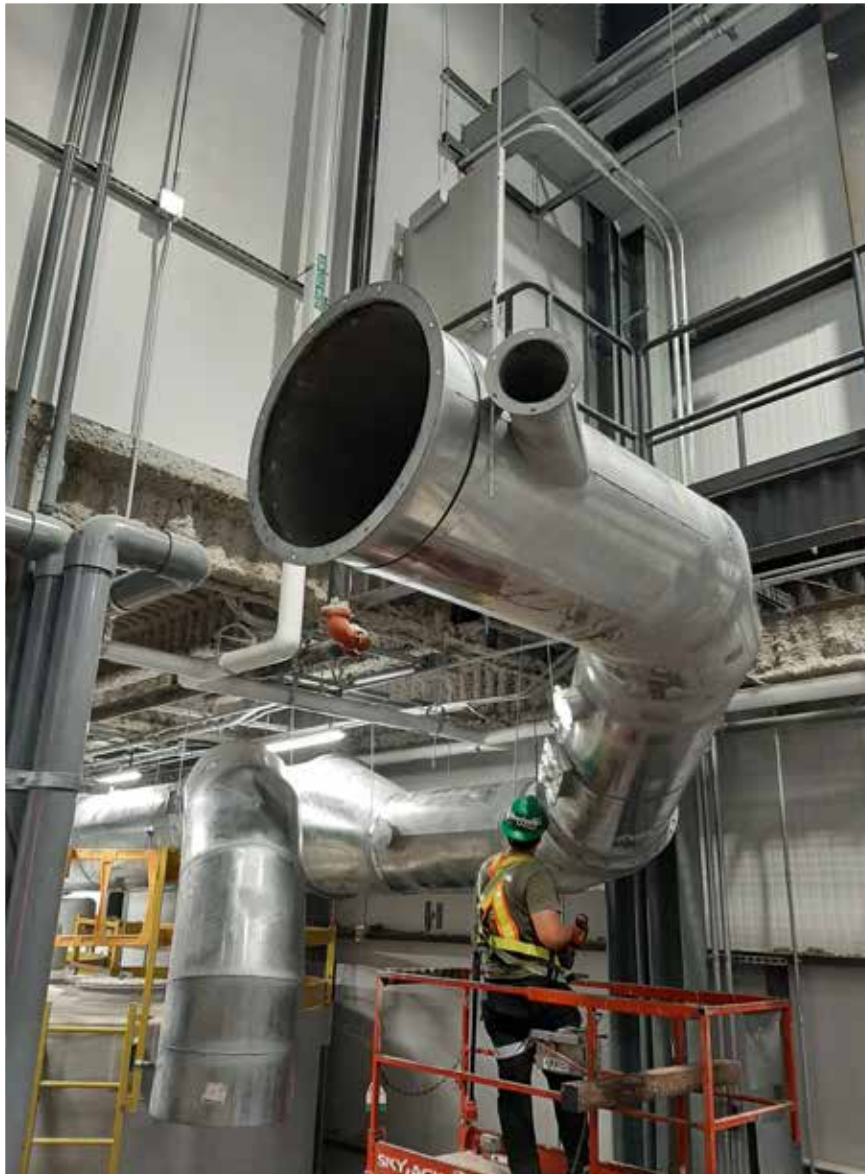
LEFT (ALL PHOTOS): Extra durable, 11-gauge steel duct was used to endure the continuous effect of sandblasting, which results from asphalt production.
