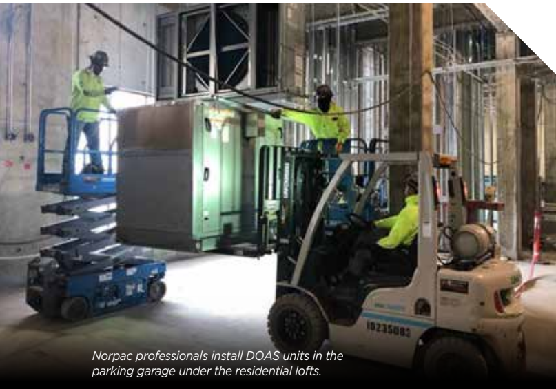
DOAS ductwork in the 32,932 square foot parking garage.
