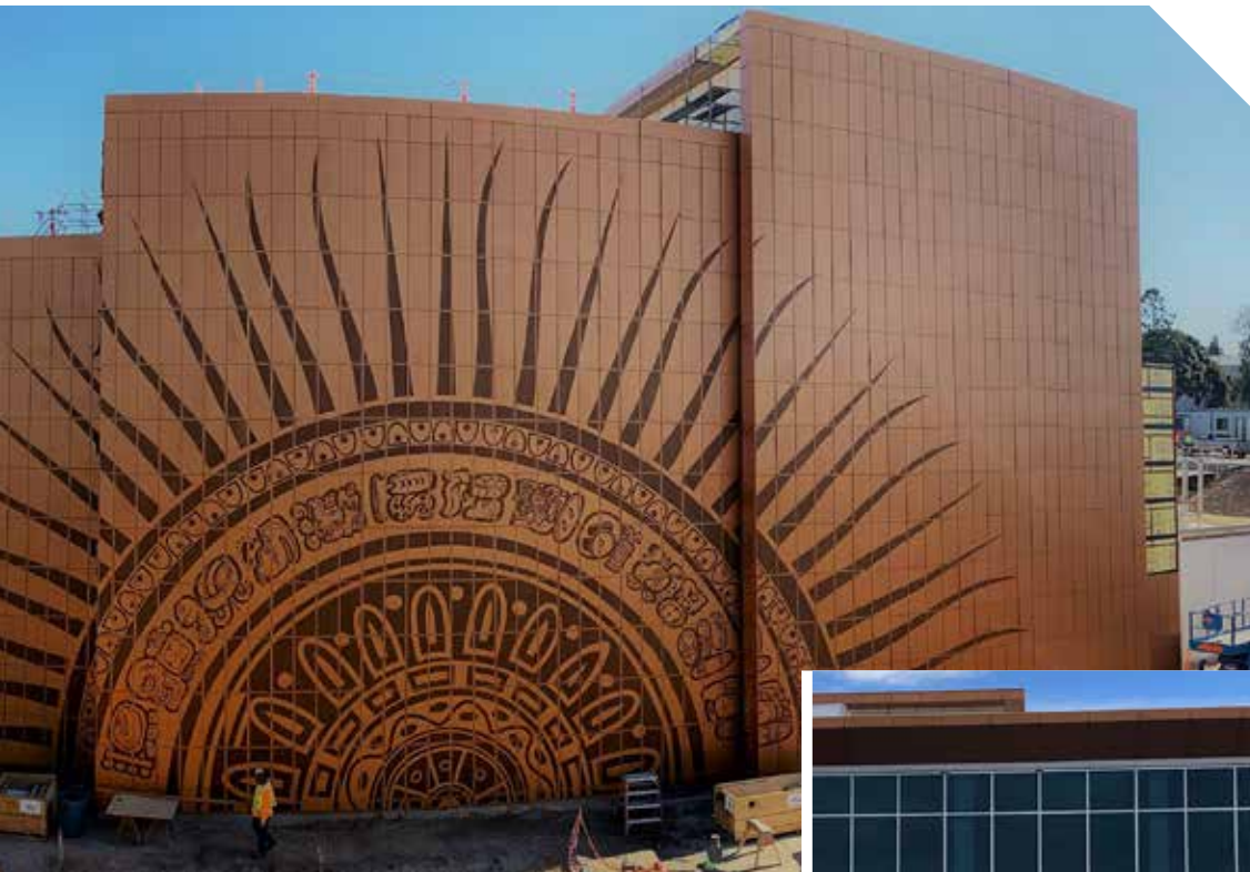
LEFT: California Sheet Metal installing .080 post finished formed aluminum soffit panels from a 65' articulating boom lift BELOW: California Sheet Metal is installing approximately 35,000 pounds of aluminum, galvanized steel, and stainless steel panels, including the perforated image of a rising sun on the exterior of the Southwestern College's new Performing Arts Center. LEFT, BOTTOM: California Sheet Metal prepping the boom lift to continue the panel install.
