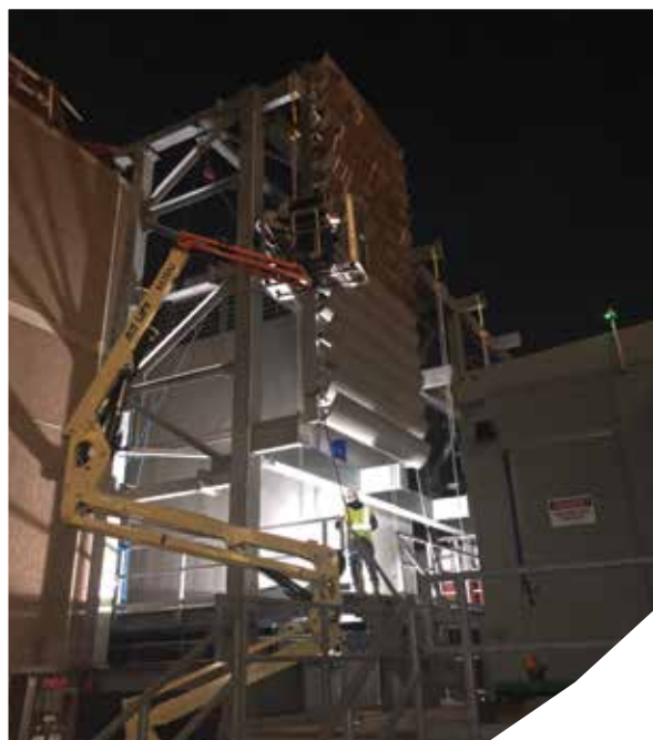
RIGHT: A night shot of the first section being installed.
