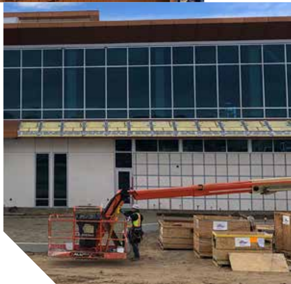
LEFT: California Sheet Metal installing .080 post finished formed aluminum soffit panels from a 65' articulating boom lift BELOW: California Sheet Metal is installing approximately 35,000 pounds of aluminum, galvanized steel, and stainless steel panels, including the perforated image of a rising sun on the exterior of the Southwestern College's new Performing Arts Center. LEFT, BOTTOM: California Sheet Metal prepping the boom lift to continue the panel install.
